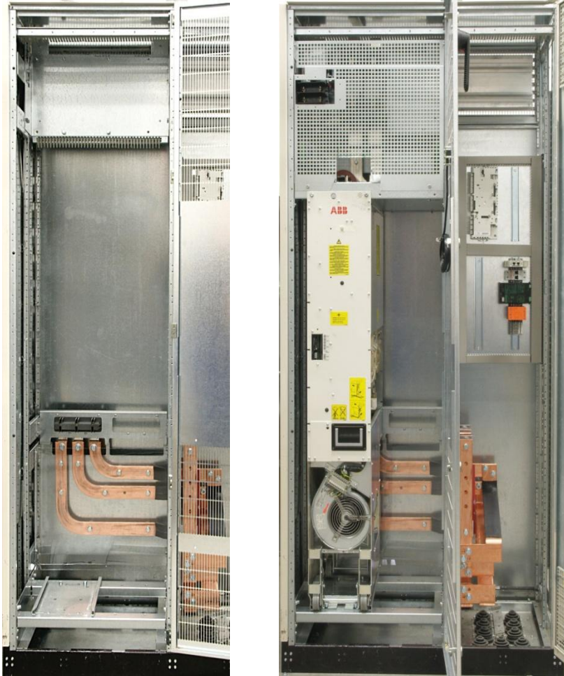
1X R8i Installation
