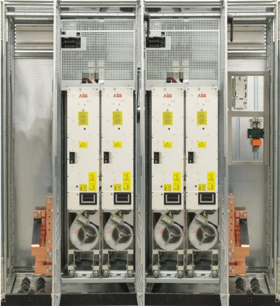
4X R8i Installation
